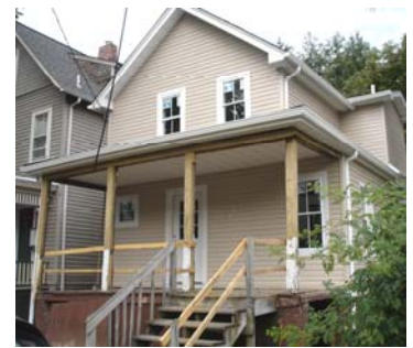
10 Miller Street, Montclair— Under rehabilitation
